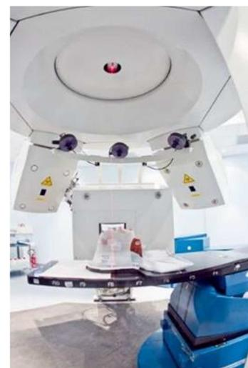
*Figure 12 – Patient positioning and position verification system in CNAO treatment room.*
